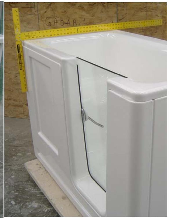
7. The final step is the installation of the front panel. This panel covers the two ends of the side panels. This step must be made with great meticulousness, in order to assure that the panel is secured and aligned in its original position. Once the panel is in place, you need to level it and the installation is complete. See figures above for panel levelling.
