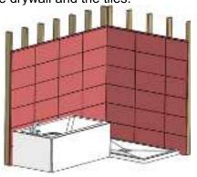
**6.** Remove the blocks, place the bathtub in its final position, and connect the drain.
