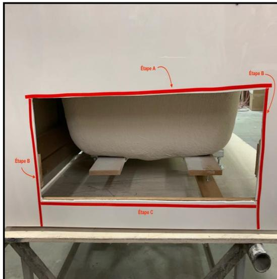
A) Install the double-sided tape horizontally over the opening. Do not exceed more than  $\frac{3}{4}$ " on each side.
