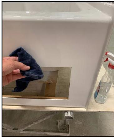
B) Clean all around the inner perimeter of the access panel, using wood alcohol.
