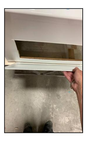
A) Apply silicone in the groove of the access panel.
